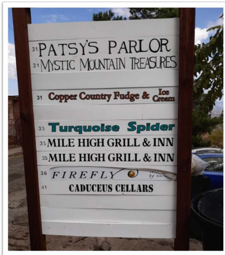
District sign on Main St. (across from Police Station) - separating panels, missing top panels, and peeling
