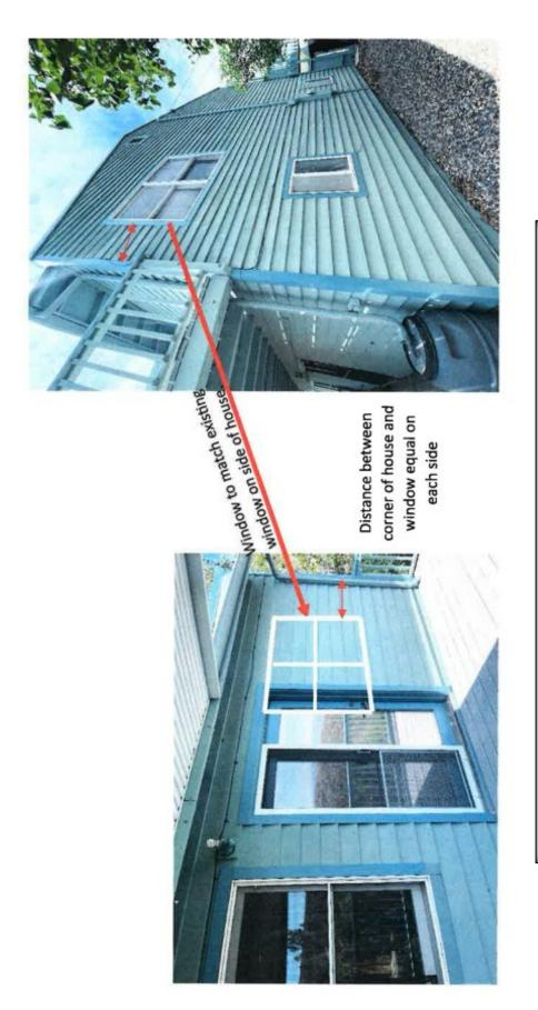
Views of the proposed work to 711 East Avenue. View is on the rear of the home (E. / S.E.) with arrows and diagrams showing the planned location of the additional window, after removal of the sliding door.
