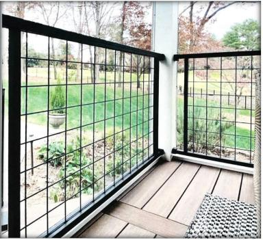
Example of the metal railing with safety wire-mesh, to prevent falling through or under the railing.
