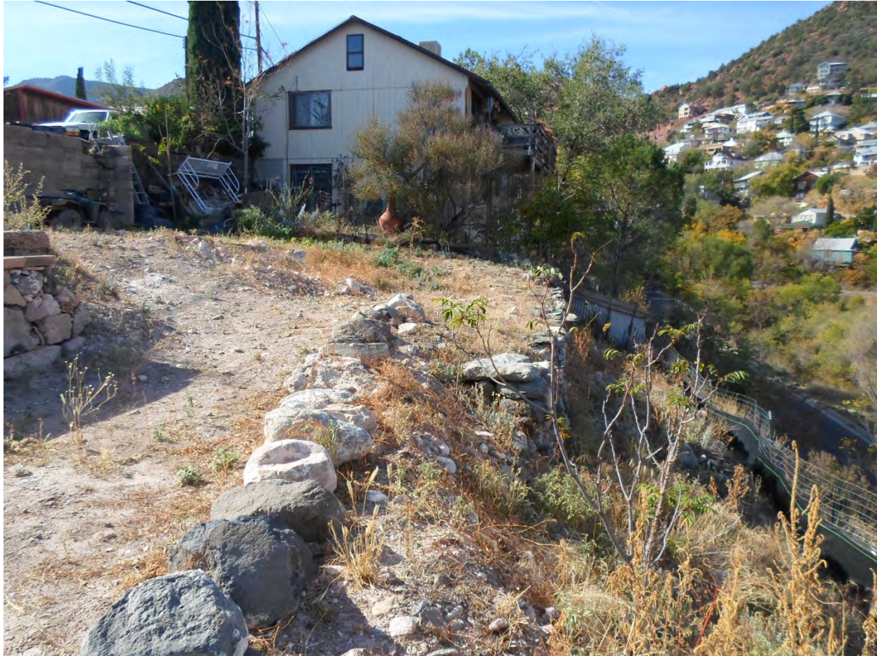
Photo 3 – View looking south along the west side of the proposed building area where a small retaining exists. The foundations for the new residence should be at least 5 feet behind this wall.
