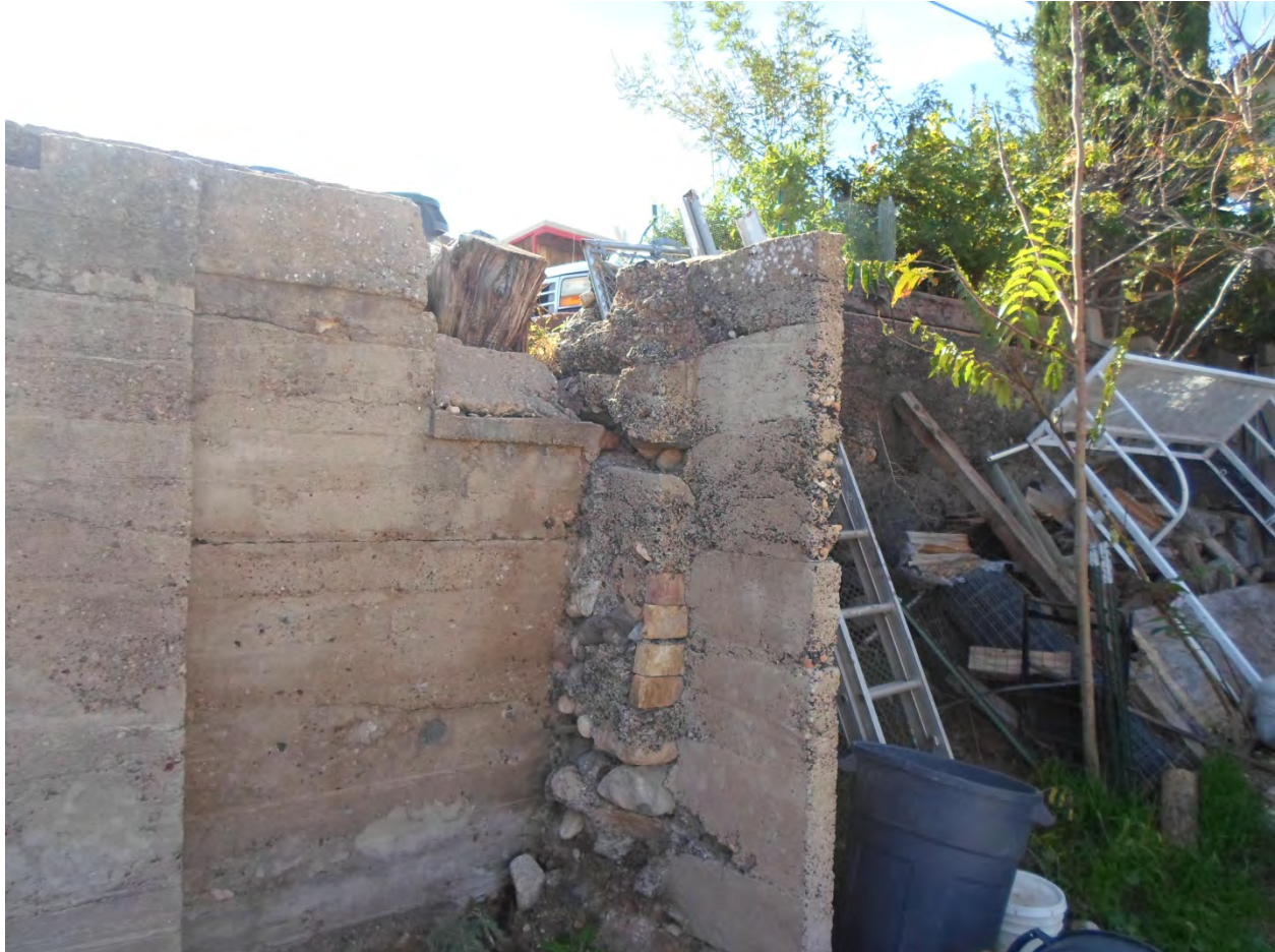
Photo 6 – View of existing retaining wall that is being undermined at the southeast corner of the lot, which is to remain. A new retaining wall will be required in front to provide support to East Avenue above the retaining wall.
