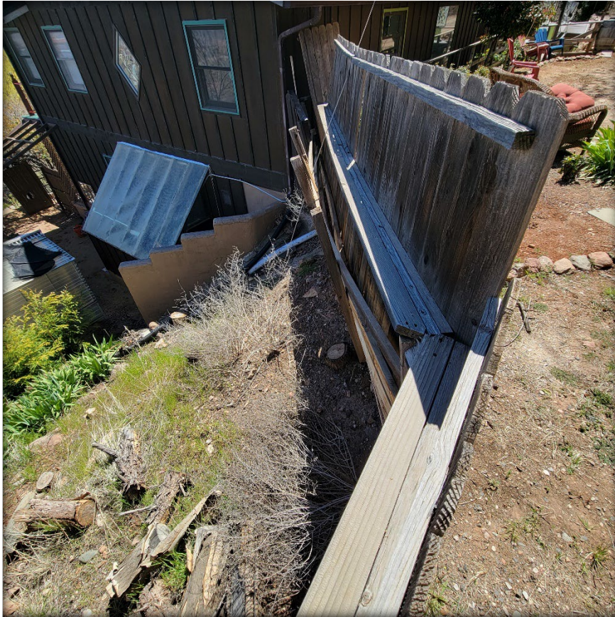
Top: Detail view showing the southern section of wooden fence and the wooden retaining wall that is failing.
