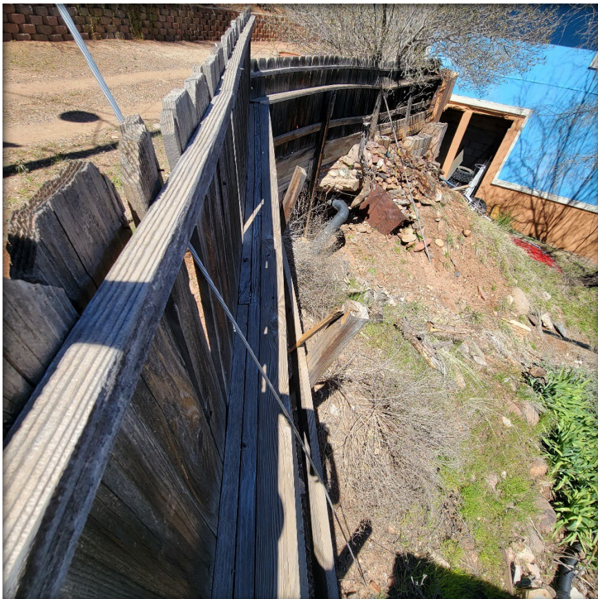
Left: Detail view along the wooden fence and retaining wall, showing previous efforts to stabilize that have failed.
