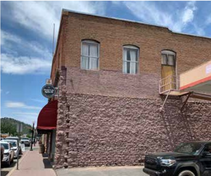
Figure 25: Mixed Masonry Types (brick and stone)
