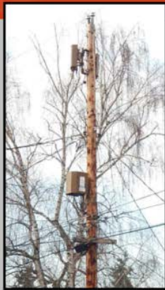
Wood Power Pole Installation in Communication Space
