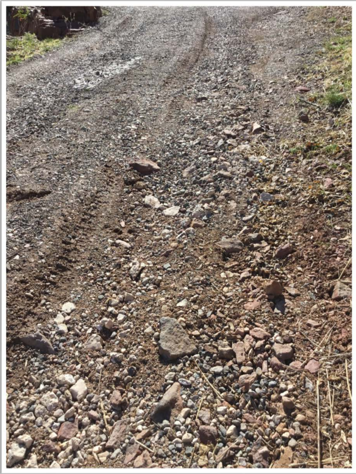
Pic showing rutted driveway and erosion
