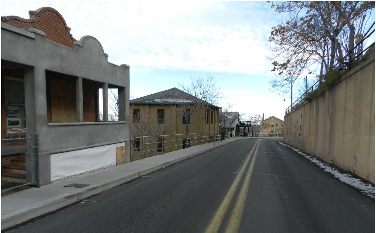
Clark St looking south
