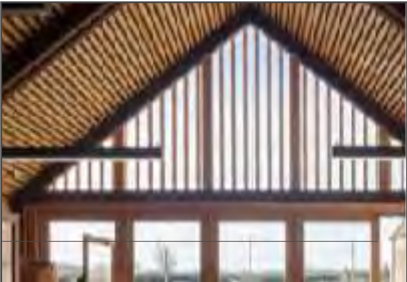
Fixed Glazing Type: Galvanized Steel Frame with A606-4 Fins and interior wood trim
