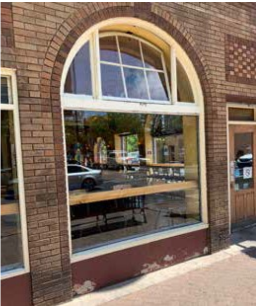
Figure 15: Preservation of Original Wood Window
