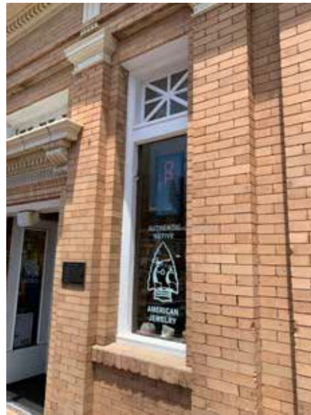
Figure 16: Vertical Window with Transom
