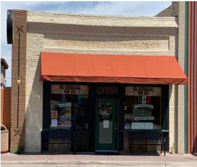
Figure 33: Awning over Storefront
