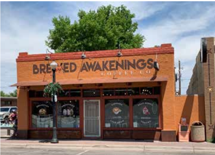
Figure 27: Painted Brick Facade (acceptable but unfinished preferred)
