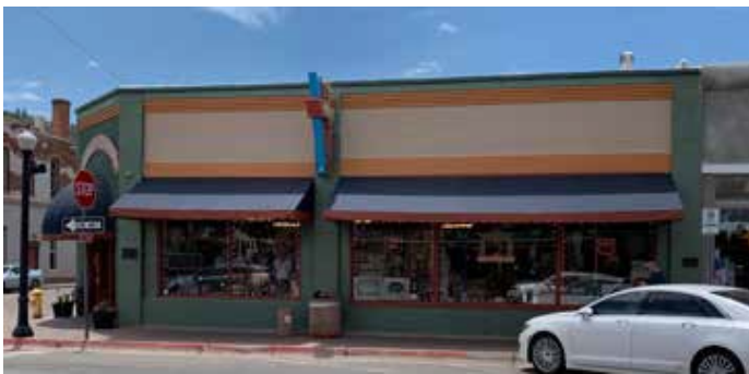
Figure 35: Multiple Awnings over Doorway and
