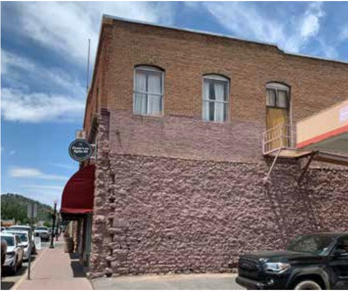
Figure 25: Mixed Masonry Types (brick and stone)
