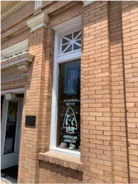
Figure 16: Vertical Window with Transom
