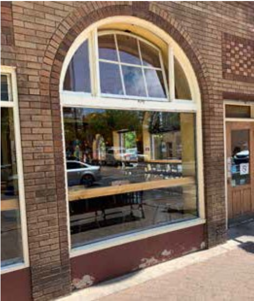
Figure 15: Preservation of Original Wood Window
