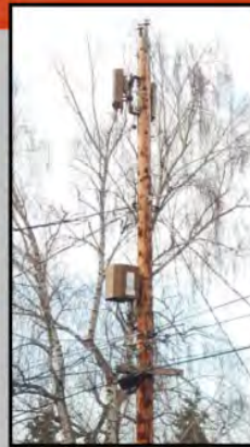
Wood Power Pole Installation in Communication Space
