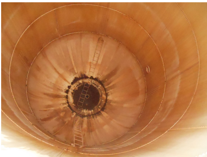
33) The wet interior bowl is in good condition. The wet interior ladder is laying in the bowl.
