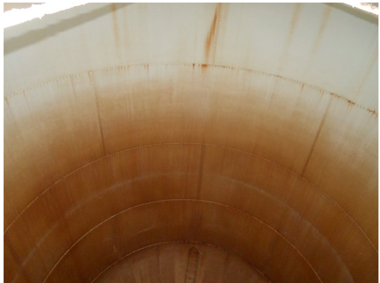
32) The wet interior sidewall is in good condition. The coating is in fair condition.
