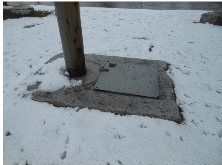
5) The riser foundation is in fair condition overall. There is a pit with a steel plate cover.
