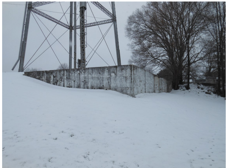
2) The tank base is surrounded by a concrete retaining wall.
