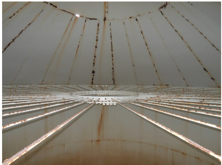
29) The wet interior roof is in good condition overall. There are small holes throughout.
