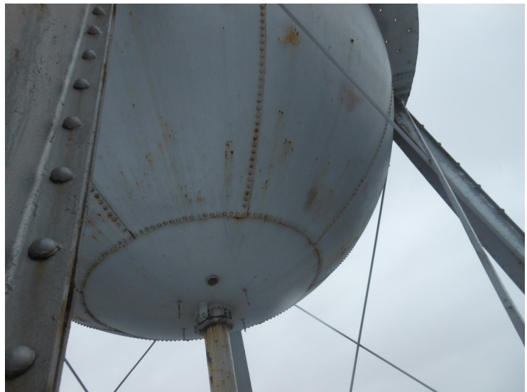
17) The bowl is in good condition overall. The coating is in fair condition.
