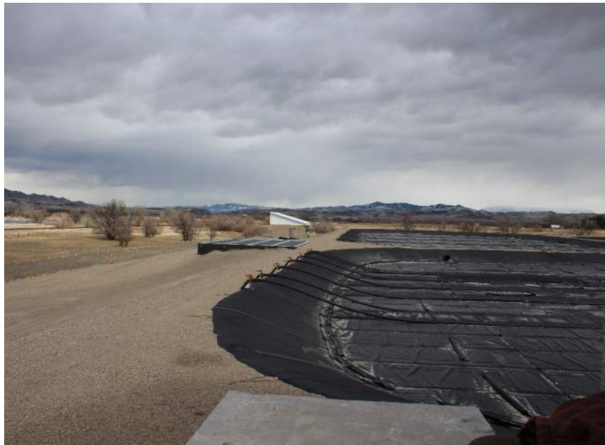
Treatment Lagoons, Polishing Reactor, and UV/Blower Building
