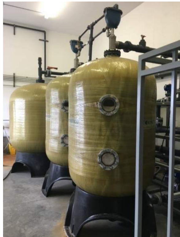
Arsenic Treatment Plant
