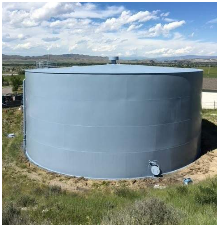
1-Million Gallon Welded Steel Water Storage Tank
