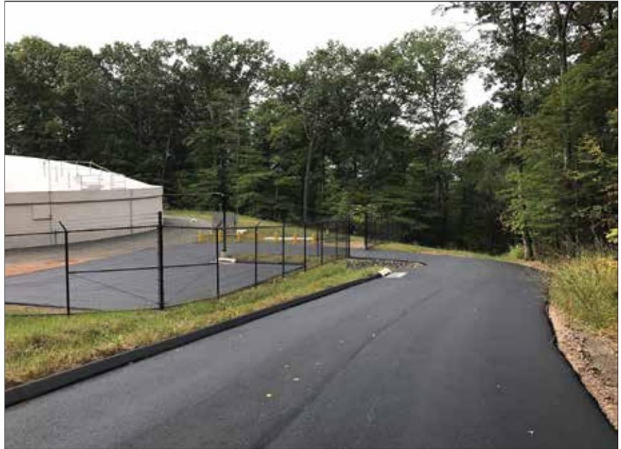
Entrance to new 1.0-million-gallon East Side water storage tank site
