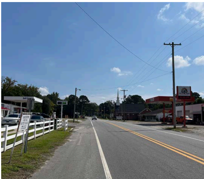
NC 124 (Green Street) functions as a commercial corridor for the Town of Macclesfield. It is a state maintained roadway that is classified as a Major Collector by the North Carolina Department of Transportation. It has two travel lanes and relatively wide shoulders through Downtown Macclesfield.
