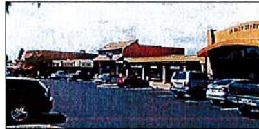
Easy Street has an eclectic mix of retail, office restaurant, and recreational uses. Providing an environment where people can shop, eat, work and play is important to creating a vibrant "downtown"; however, the physical placement of these uses is just as important in order to promote and maintain an active streetscape.
