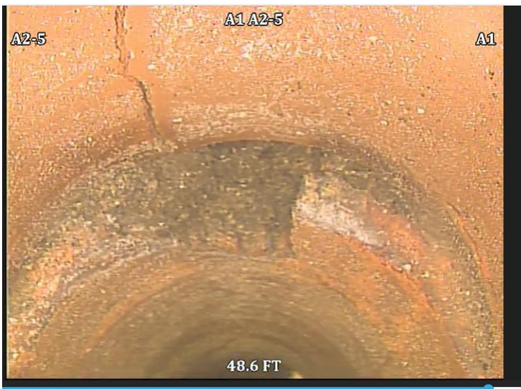
Picture of A1-A2.5 sewer line crack.
