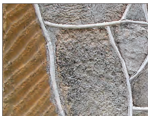
Section of a giraffe rock wall with narrowly beaded mortar joints painted white. It includes some nice ripplestone. Photo by Primas.
