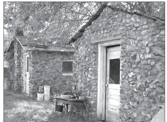
Above J. D. Stanton built Spring Valley Camp on Route 66 east of Hazelgreen in the 1920s using rubble rock construction for his tourist cabins. Right While the wooden doors were rotting in 2007, the rock walls were fine.
