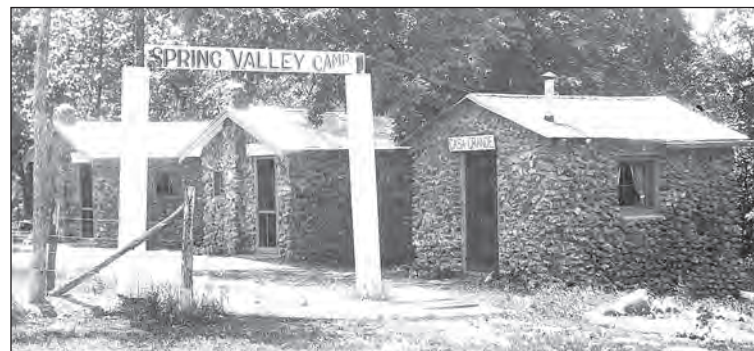
Above J. D. Stanton built Spring Valley Camp on Route 66 east of Hazelgreen in the 1920s using rubble rock construction for his tourist cabins. Right While the wooden doors were rotting in 2007, the rock walls were fine.
