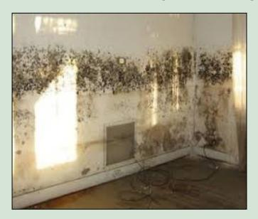
If your house does not have eaves, it is especially prone to having wet walls. In the 40's, homes were often built without eaves. Gutters were installed where the wall and roof intersected, allowing rain to easily pass behind the gutter and drip directly into the wall cavity, causing mold and mildew and making the home harder to heat.
