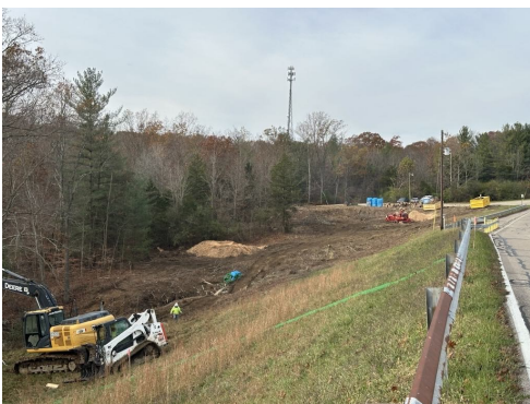
Clearing the downslope area
