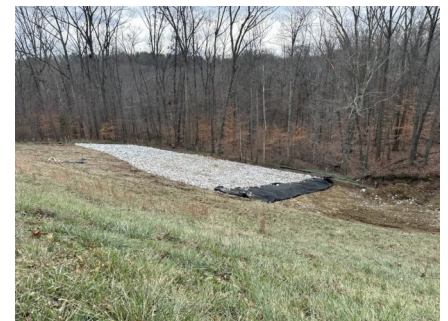
Rip-rap installed east of the spillway
