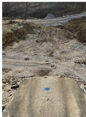
Concrete removed from old spillway
